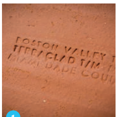
1 A detail of a Boston Valley rain screen panel. 2 Raw clay arrives from within 500 miles of the plant and is then mixed to create specific colors. 3 Each “supersack” of clay weighs about 2,200 pounds. 4 The formed clay panels are baked at 2,100 degrees Fahrenheit for more than 24 hours. 5 Each panel is checked for color accuracy with a spectrophotometer. 6 Finished panels are packed into protective crates and shipped to the job site.
