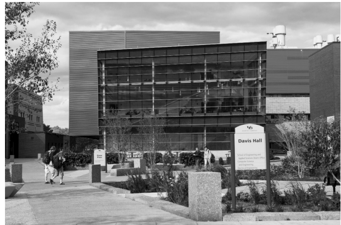
Davis Hall, on UB's North Campus
